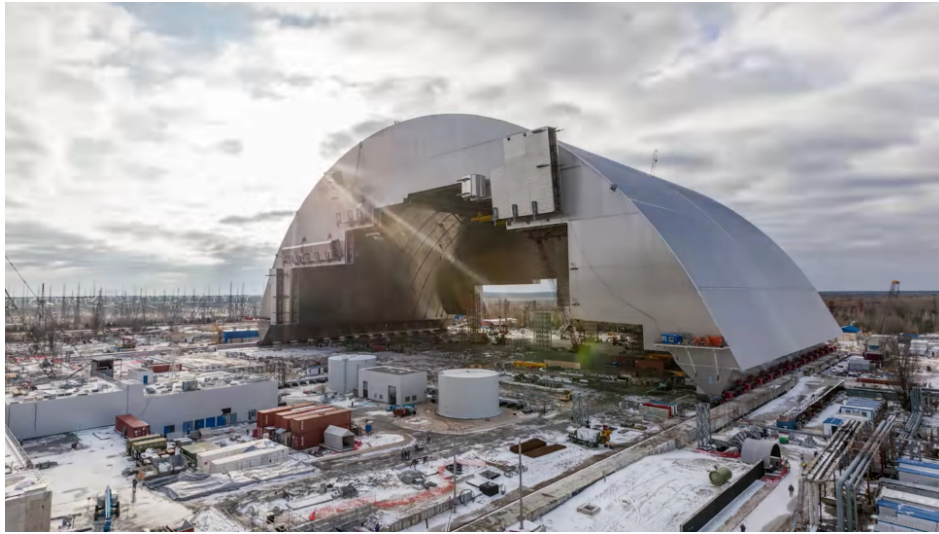
Fig.3.1: The Chernobyl New Safe Containment, standing at 150m high, with an arch span of 275m, and weighing 31,000 tonnes.
