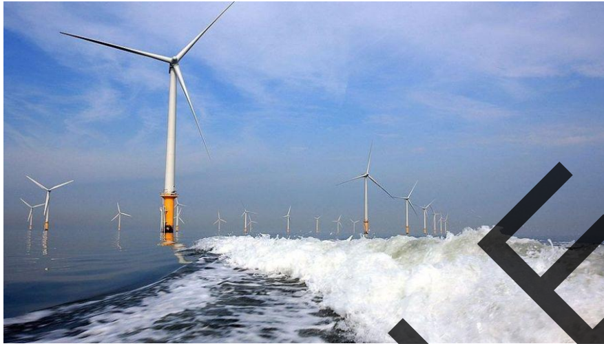
Figure 1.3: Burbo Bank Offshore Windfarm in Liverpool
