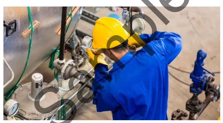
Where the device examined follows a sequence, the operation should be checked to ensure all ancillary devices, such as limit switches, are operating. The time to perform sequences may be worth recording as a lengthening of sequence times may indicate a possible developing fault due to, say, leakage in a cylinder.
